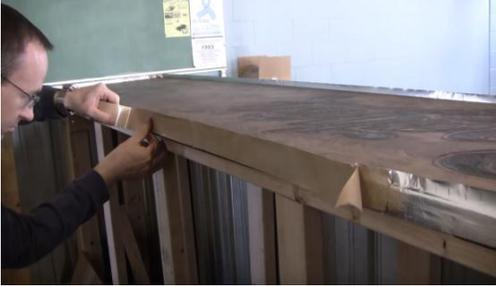
**Note:** Un-level surfaces can cause resin to pool and ultimately use more resin. In some extreme cases, a uniform coating will not be achieved resulting in thin and thick areas. Pooling resin will create pressure on the tape that can cause the tape to release prematurely. To prevent this, apply tape to a clean surface and press firmly to form a good bond. A supporting piece of trim could also be applied on the outside perimeter to support the tape.
