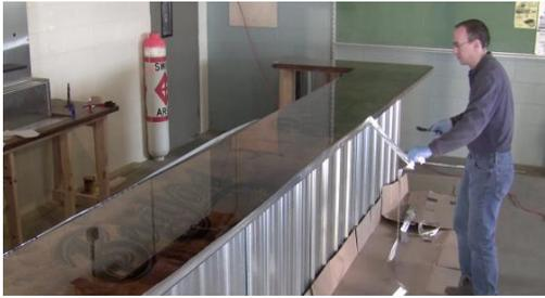
**Aluminum Tape:** If Aluminum tape was used, the tape can be removed when resin has thickened slightly, but still flows. Again, use a brush or foam applicator to assist in uniform coverage and removal of excess resin if needed.
